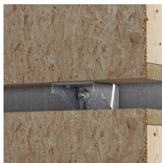
Brackets set below, on slab edge
