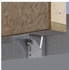
Bracket below, in the middle of concrete
